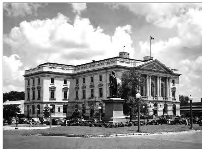
A pre-1950s view of the federal building showing the wing added in 1917, during the building's first major renovation.
