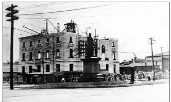
Macon's second federal building and courthouse goes up, circa 1906-1908.
